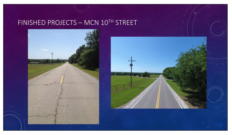
This 9-mile project was completed by the Muscogee (Creek) Nation in Hughes County, Oklahoma. It involved installation of new guardrail, patching and an asphalt overlay on a county road.
